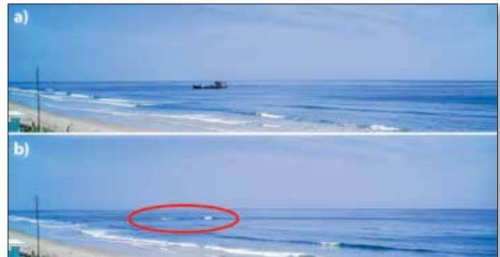
Figure 3. a) The USACE hopper dredge Murden placing sediment in the near-shore, and b) the waves breaking over the newly placed material.
