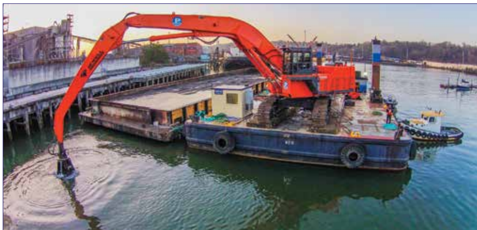
Long reach Hitachi 1200 excavator placing granularly activated carbon (GAC) in the Duwamish Waterway – Photo courtesy of Pacific Pile & Marine
