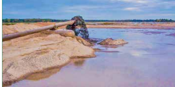
Hydraulic discharge pipe placing dredged material at Detroit District's Cat Island project in Green Bay, Wis. (U.S. Army Corps of Engineers, Detroit District photo).
