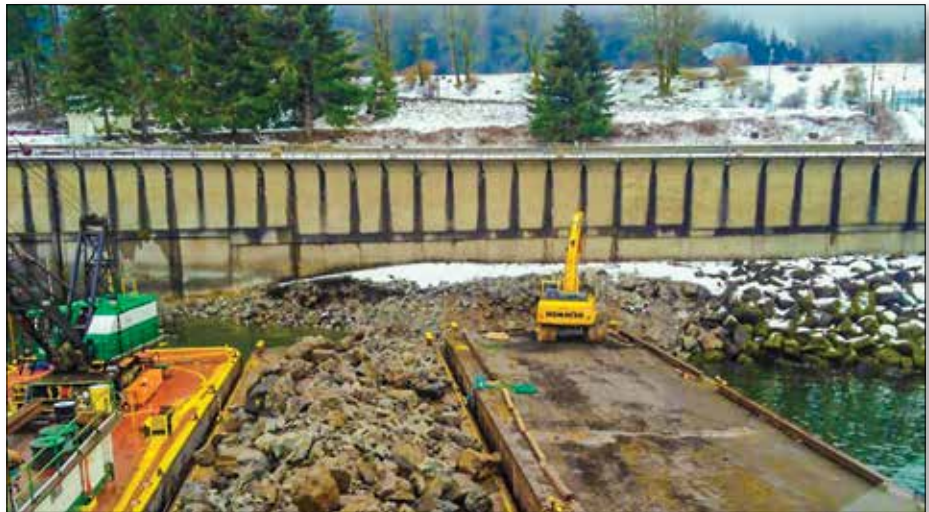
Figure 5. Dredge and Excavator working on demolition
