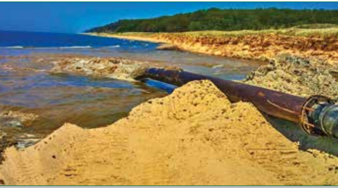
Placement of dredged material in near shore beach nourishment site in Muskegon Harbor, Mich. This material is dredged from the entrance channel of the Muskegon outer harbor (U.S. Army Corps of Engineers, Detroit District photo).
