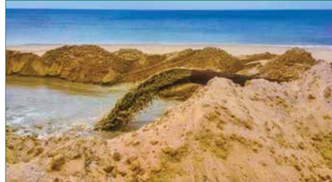
Dredged material placement south of the south pier at St. Joseph Harbor, Mich. Material is dredged from the entrance channel for placement in the near shore beach nourishment site (U.S. Army Corps of Engineers, Detroit District photo).
