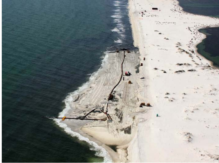
Figure 1. Swash zone berm being built at Perdido Key, Florida in 2012 (Photo provided by SAM).
