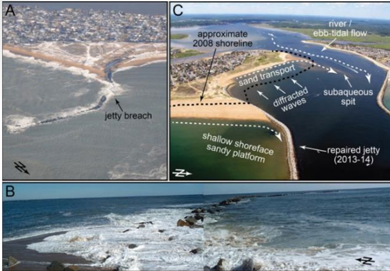
(A) Refracted northeast storm waves propagate through a breach in the South Jetty during high tide. (B) Merged panoramic of waves delivering sediment through the breach in the South Jetty to proximal Reservation Terrace. (C) Aerial view of northern Plum Island following jetty repair showing erosional beach of Reservation Terrace and growth of oceanfront beach south of Merrimack River Inlet South Jetty. (Hein, Fallon, Rosen, et al., 2019)
